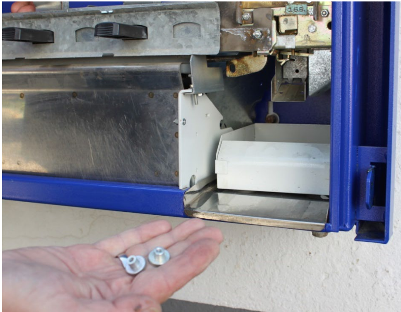
Remove two screw nuts
